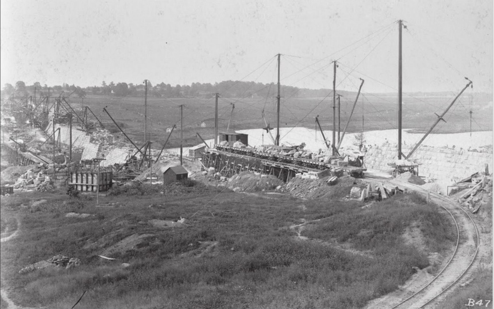
Historic photo of temporary railroad used in construction of the Boonton Dam. Credit: Courtesy of Boonton Historical Society
