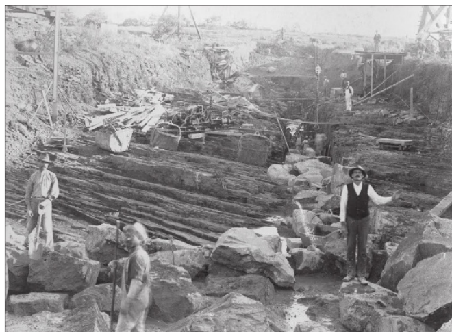
Dam workers around 1900 standing on shale foundation before the core of the dam was laid. Credit: Courtesy of Boonton Historical Society
